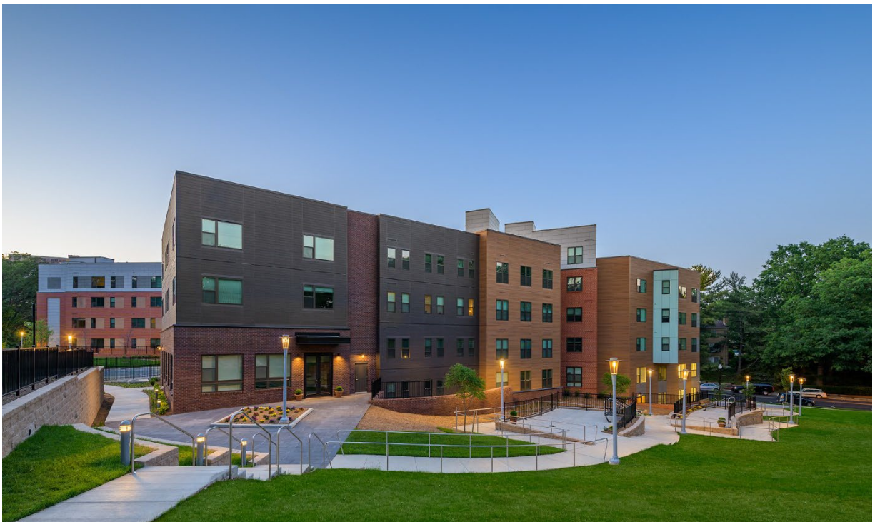
St. James Plaza (93-Unit Affordable Housing Building in partnership w/ St. James Methodist Church) (Alexandria, VA) (Developer: AHC / Architect: Cunningham | Quill Architects / Photographer: Allen Russ)
